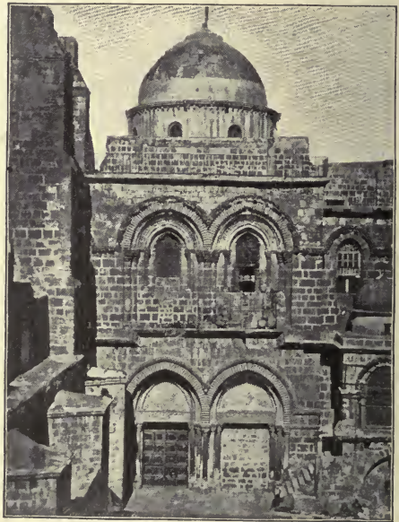
CHURCH OF THE HOLY SEPULCHER Present condition
